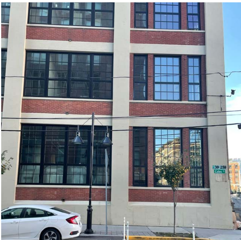
PHOTO OF NEW WINDOWS & RESTORED CONCRETE (CORNER OF COLES AND 16 TH STREET)
