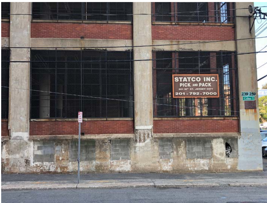
PHOTO OF NEW WINDOWS & RESTORED CONCRETE (CORNER OF COLES AND 16 TH STREET)
